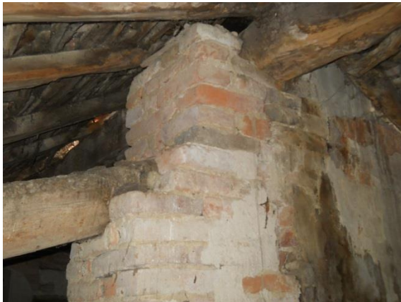
Figures 198-199. Seismic events 2012 in Emilia_ damage suffered by wall 14 on the second floor
