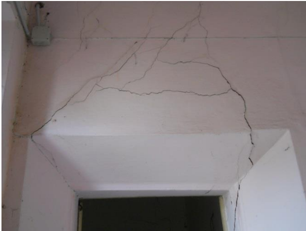
Figures 196-197. Seismic events 2012 in Emilia_ damage suffered by wall 14 on the first floor
