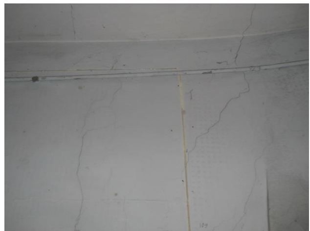
Figures 194-195. Seismic events 2012 in Emilia_ damage suffered by wall 14 on the ground floor
