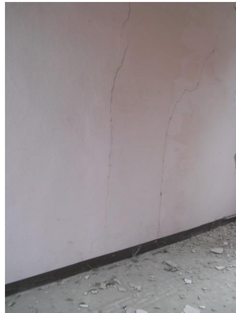
Figures 196-197. Seismic events 2012 in Emilia_ damage suffered by wall 14 on the first floor
