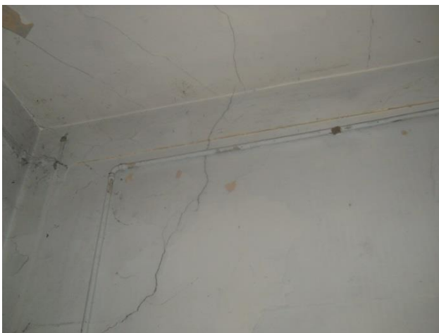
Figures 194-195. Seismic events 2012 in Emilia_ damage suffered by wall 14 on the ground floor
