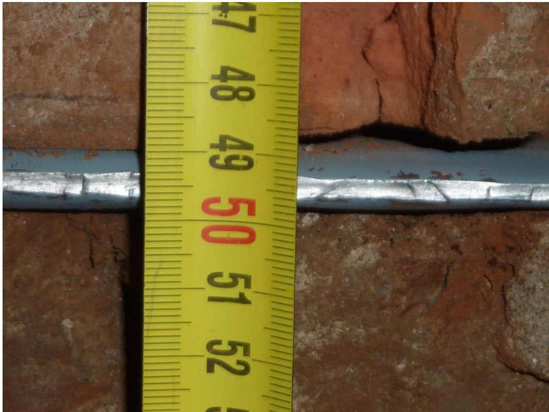
Figure 95. Double flat jacks test
