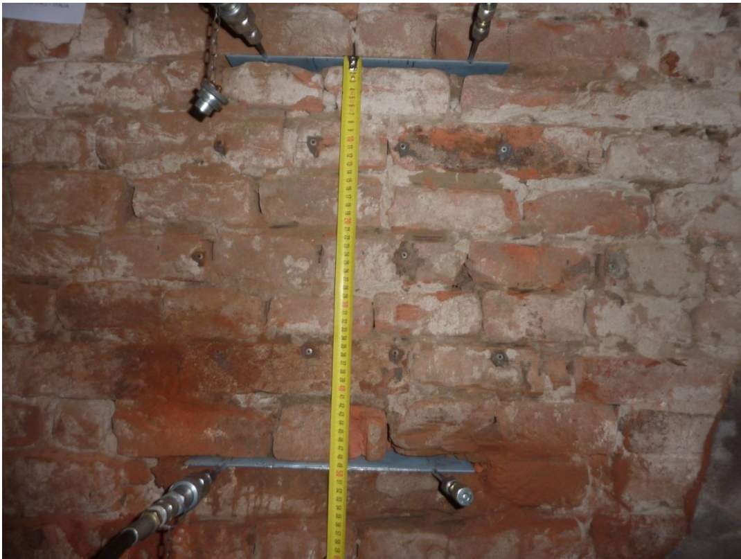
Figure 94. Double flat jacks test
